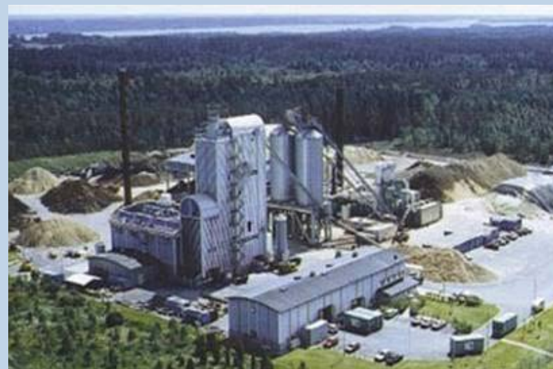
10 MW wood residue CHP plant (Vaxjö, Sweden) which uses gasification
