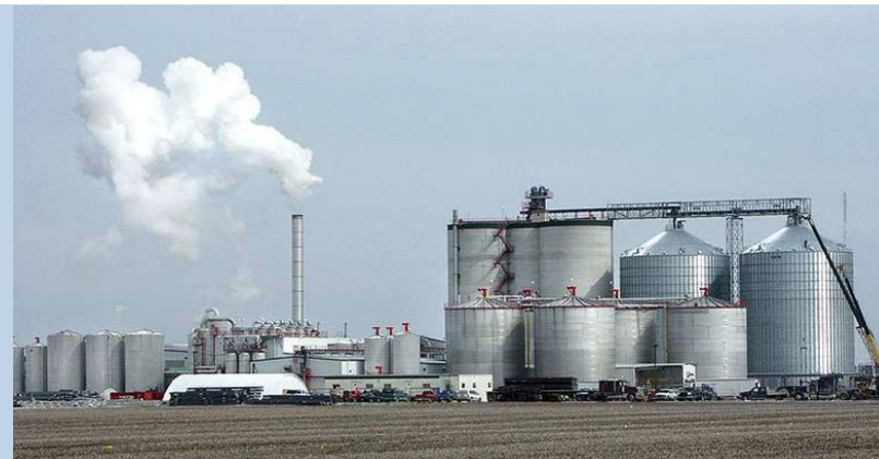
280 MW corn bioethanol plant (West Burlington, USA)
