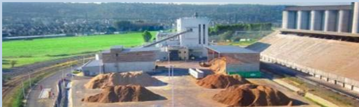
9 MW wood residue CHP plant (Rouen, France) which uses combustion to generate energy
