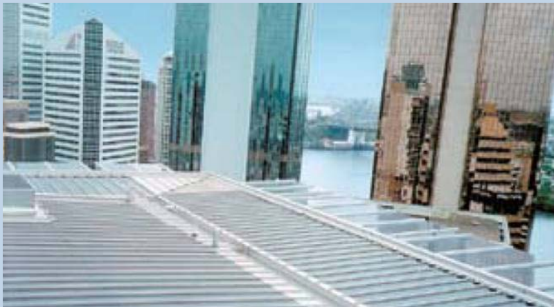
Flat stainless steel roof with integrated amorphous PV cells
