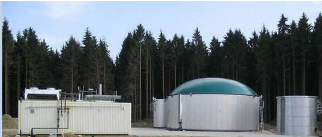
Frankfurt Hahn Airport's co-generation plant
