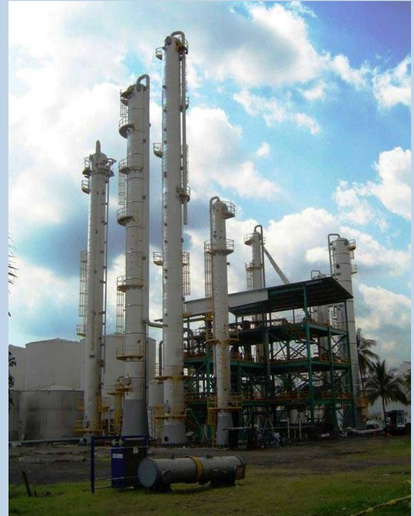
Stripper/Rectifier, fully assembled, fabricated using 304 stainless steel
